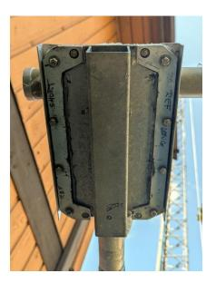
The reconditioned fibreglass tubes were ready to be attached to the EHUs. New bug screen end caps were ordered from SteppIR and installed.
